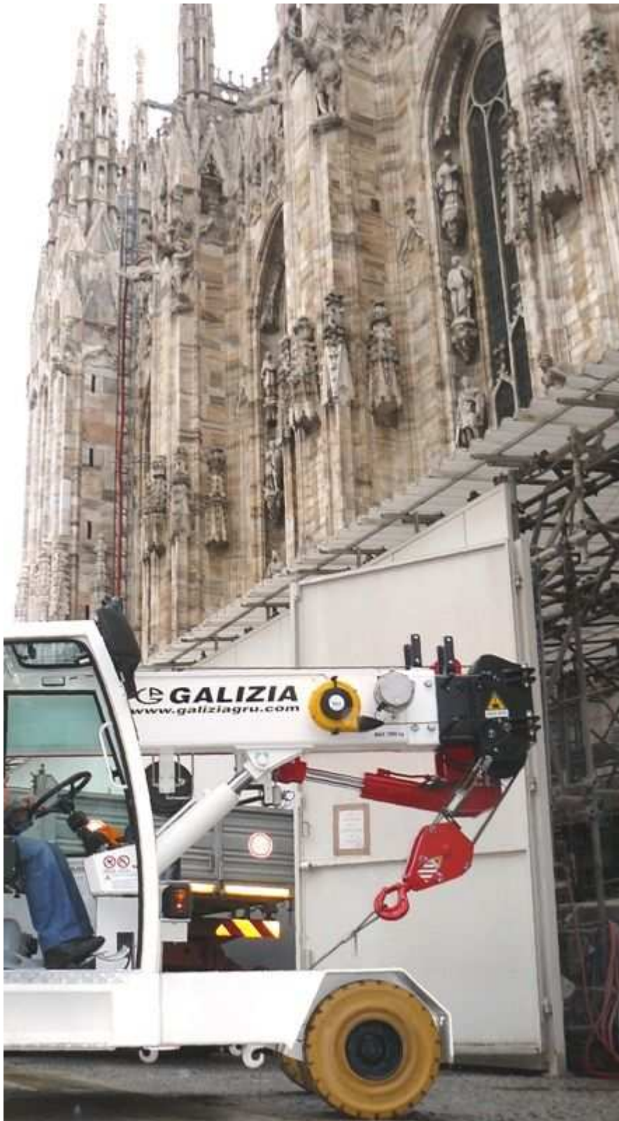
The crane working in the building yard near the Duomo
